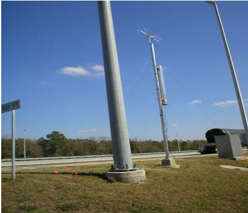
Figure 2.7 Typical assembly of a vehicle scanner tower, strapped to an existing height-detector pole.
